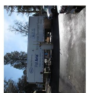
tunnel AWS a safe The Pall Trailer is known as the Alternative Water Supply (AWS) treatment plant. The AWS was installed in 2008. It is capable of producing 600 gallons per minute of treated water drawn outage, or emergency situation, the AV treatment plant is capable of providing a s drinking water supply to all GCSD customers. Mountain Lake. During a The Pall Trailer is known as the Pine from
