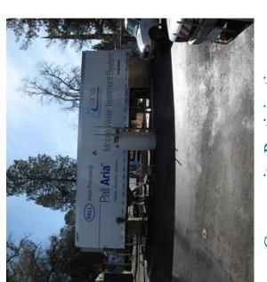
tunnel AWS a safe The Pall Trailer is known as the Alternative Water Supply (AWS) treatment plant. The AWS was installed in 2008. It is capable of producing 600 gallons per minute of treated water drawn outage, or emergency situation, the AV treatment plant is capable of providing a s drinking water supply to all GCSD customers. Mountain Lake. During a Pine from
