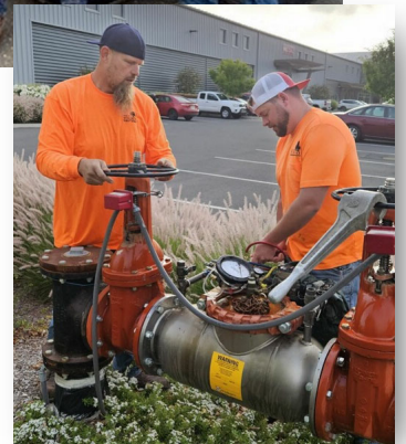
Left: Windsor Water Operations staff conducts backflow testing.
