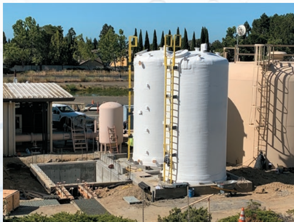
Figure 1 New Sodium Hypochlorite Tanks
