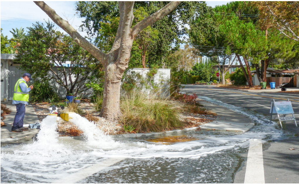
Flushing water mains provides the highest water quality possible.
