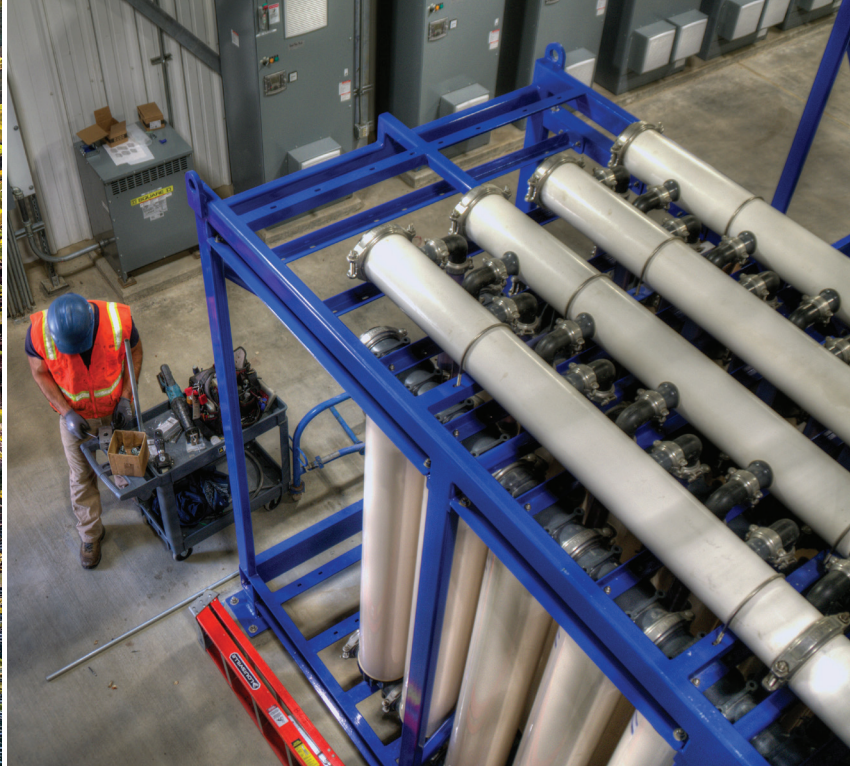
Ultrafiltration modules, like the one shown above, remove parasites, bacteria, and viruses from the water.
