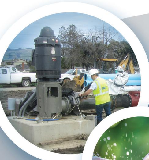
Connecting the last piece of piping for well operation at McLaughlin Station
