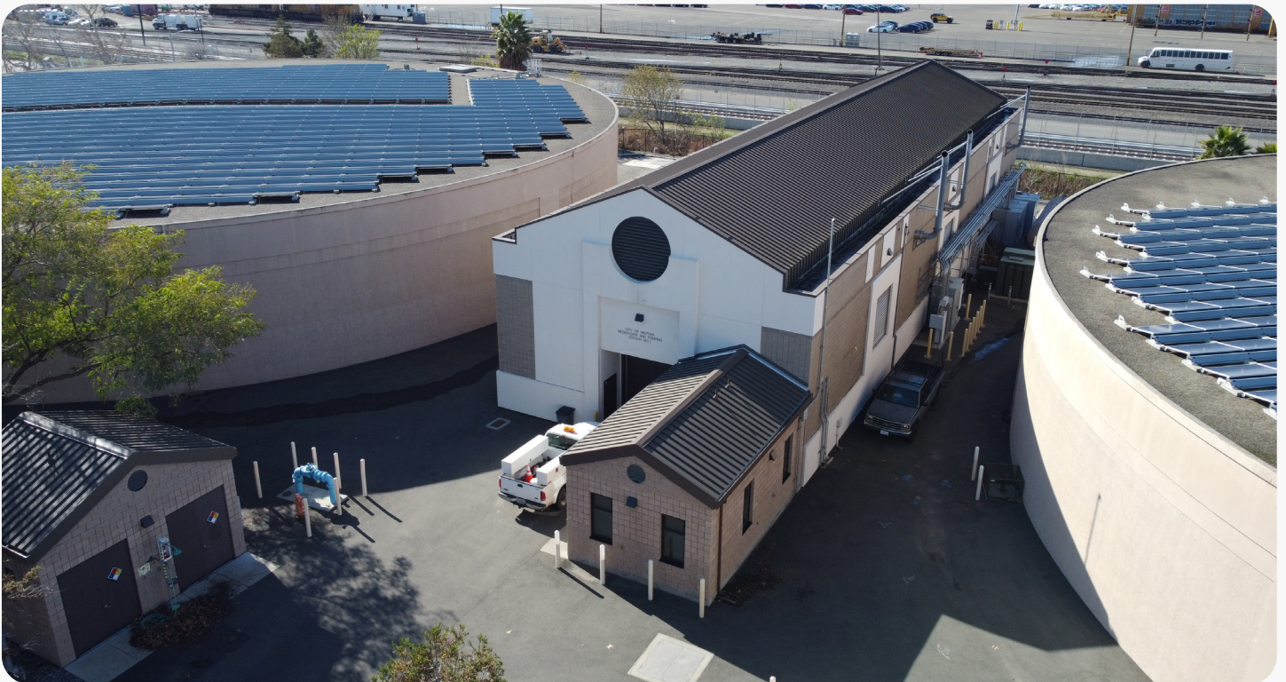
Gibraltar Pump Station/Reservoirs - The City's Gibraltar Water Facility stores, pumps, and regulates the pressure of both SFPUC and Valley Water supplies.
