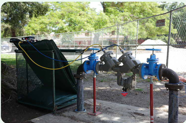
Backflow Prevention Assembly - One of over 2,300 backflow prevention assemblies in the City.
