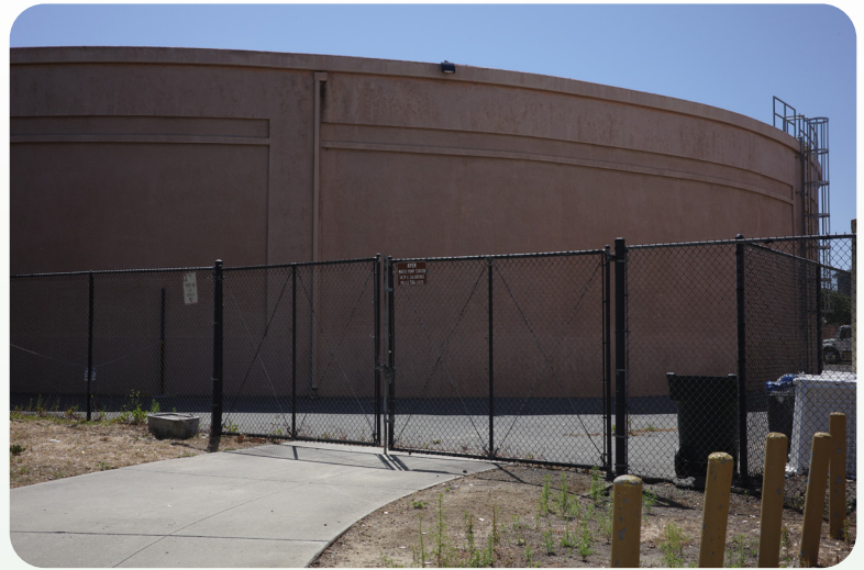
Ayer Pump Station & Storage Reservoir - Ayer Pump Station & Storage Reservoir, located along E. Calaveras Blvd. serves customers with water from SFPUC.
