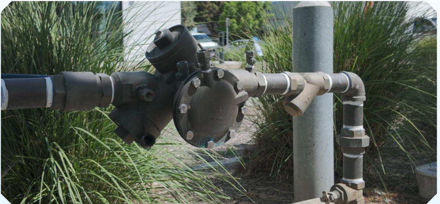
Backflow Prevention Assembly - One of over 2,200 backflow prevention assemblies in the City.
