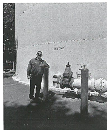
Picture of Menlo Park Fire Captain K. White standing in front of our 350,000-gallon water storage tank F.D. CONN. (Fire Department Connection).
