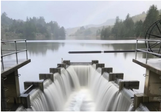
Pilarcitos Reservoir Spillway
