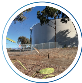
12 Closed Steel Tanks
