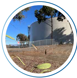
12 Closed Steel Tanks
