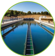
Coagulation, Flocculation & Sedimentation
