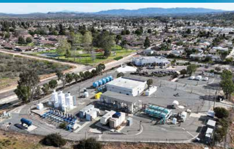
The Mission Basin Groundwater Purification Facility uses reverse osmosis to treat local brackish groundwater extracted from the Mission Basin aquifer.
