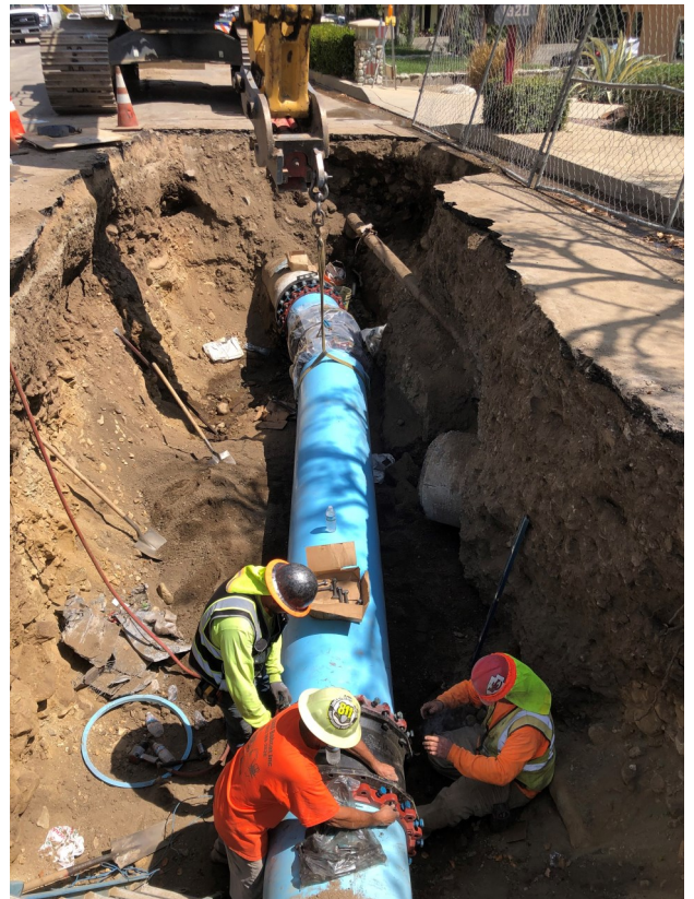
Reservoir 9 Waterline Replacement
