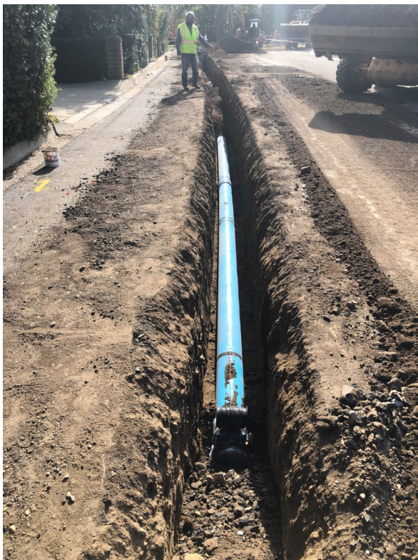
Euclid Crescent East Domestic Pipeline Replacement
