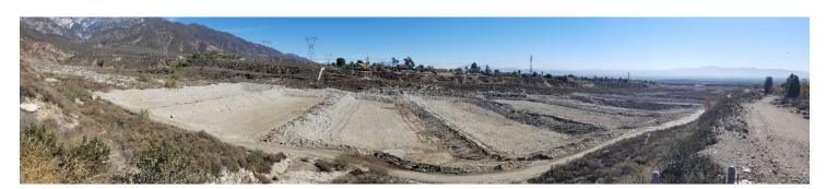
Above, the Crosswalls before the rain. Below, after the rain came in April 2020. Crosswalls working like they are designed to do which is to trap and store canyon flow, allowing it to percolate into and recharge the groundwater.
