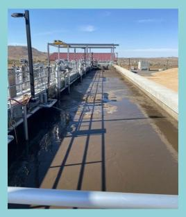
HDWD's wastewater reclamation facility was constructed over an 18-month period. Substantial completion was reached in fall 2019, and the facility began receiving local effluent in November 2019 and discharging clean water into its percolation ponds in February 2020. This reduced the number of septic systems and the threat of nitrate infiltration to the aquifer.
