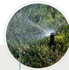
**Run each irrigation zone individually** on the 'manual' cycle, and check for broken sprinklers heads. Replacing broken sprinklers can save about 3,000 gallons of water.
