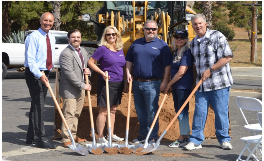
The Board of Directors and General Manager of the Yucaipa Valley Water District celebrating the groundbreaking of the Calimesa Recycled Water Pipeline Project.
