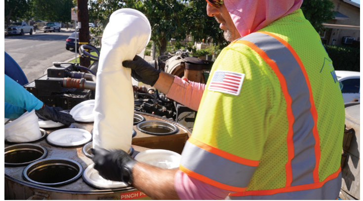
Workers inserting clean filters into the NO-DES system before another round of flushing.
