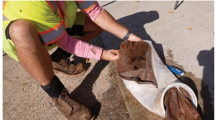
Used filters show how much sediment was able to be removed from mainlines.
