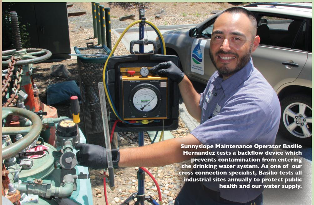
**Sunnyslope Maintenance Operator Basilio Hernandez tests a backflow device which prevents contamination from entering the drinking water system. As one of our cross connection specialist, Basilio tests all industrial sites annually to protect public health and our water supply.**
