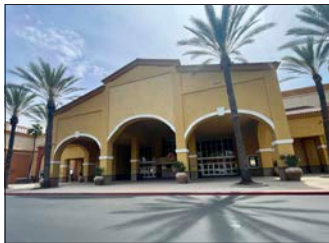
Costco has submitted plans to build a 160,000-square-foot store at Foothill Ranch Towne Centre in Lake Forest, where it would demolish a former movie theater that closed in 2024. SAMANTHA GOWEN — STAFF
