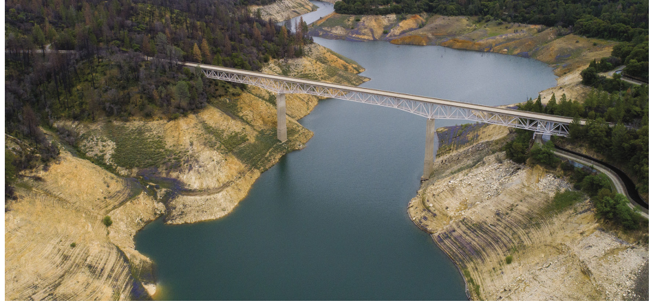
Enterprise Bridge over a section of Lake Oroville. In May 2022, water levels at Lake Oroville have dropped to 55 percent of its capacity. (Image provided courtesy of California Department of Water Resources)
