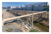
Northern Santa Fe Corporation (BNSF) railroad and across a flood control channel to provide a redundant water supply source to approximately 200 customers south of Orangethorpe Avenue.
