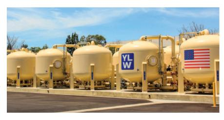
Located at our existing headquarters in Placentia, the PFAS Treatment Plant uses an IX treatment system of highly porous resin that acts like powerful magnets that adsorb and hold onto contaminants. It consists of 6 pre-filters, 22 IX
