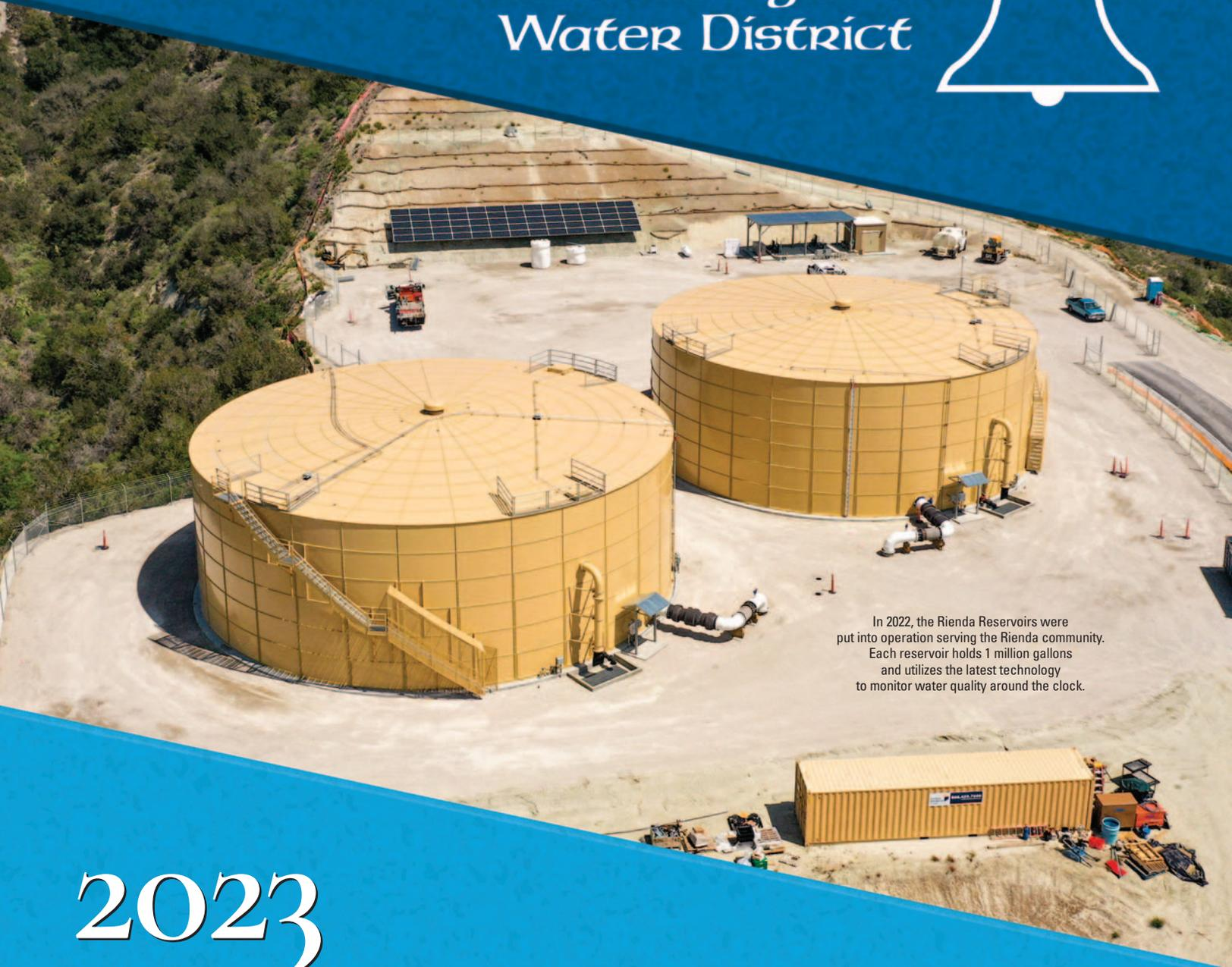
In 2022, the Rienda Reservoirs were put into operation serving the Rienda community. Each reservoir holds 1 million gallons and utilizes the latest technology to monitor water quality around the clock.
