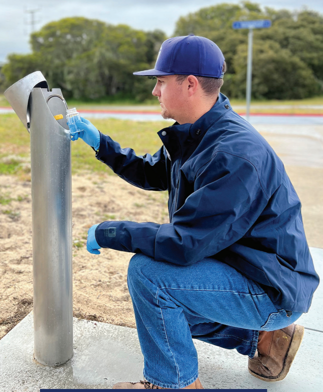
Operator collecting a water sample at an upgraded sample station.
