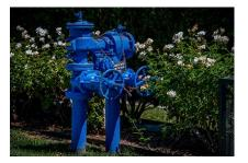
An integral part of cross-connection control measures are Backflow Prevention Assemblies (BPA). BPAs are critical components in plumbing systems to prevent the reverse flow of water from a customer's property into the clean water supply. The type of BPA required to be in place at a customer's property is based on various factors used to assess the degree of hazard to the public water supply.
