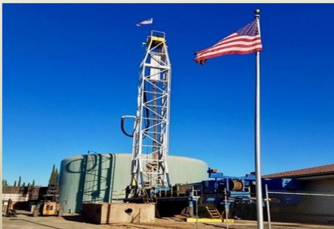
*South Montebello Irrigation District has finished the drilling of the new well at the office located on bluff road in March 2020. The next steps for the well is to construct the well motor, generator and connecting it to the system mains before putting the well in operation.*
