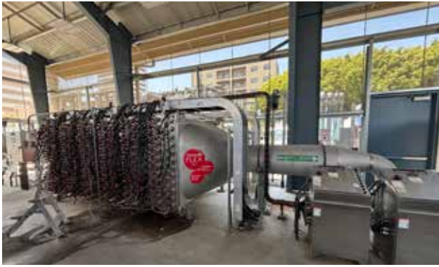
Ultraviolet Light Advanced Oxidation Process Removes Industrial Contaminants from the Olympic Well Field.
