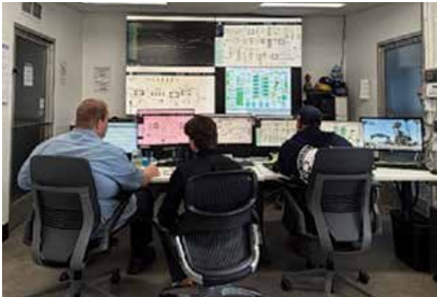
Operators Monitor Water Quality, Treatment Processes, and Production 24/7 at the Arcadia Water Treatment Plant.
