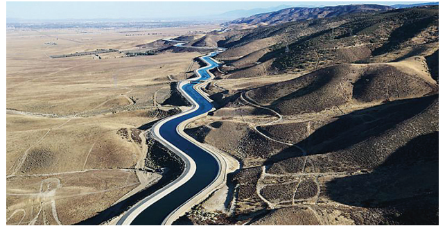
The California Aqueduct.
