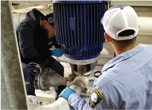
Operators performing repairs on RO Equipment.
