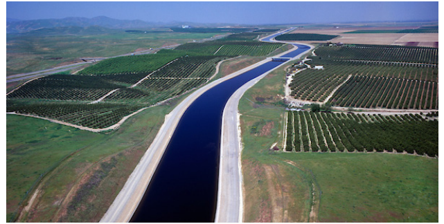
Photo of the California Aqueduct by the Department of Water Resources.
