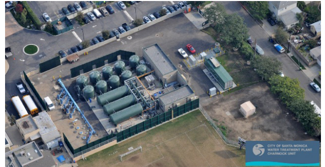
Charnock Well Field and Charnock Treatment Plant
