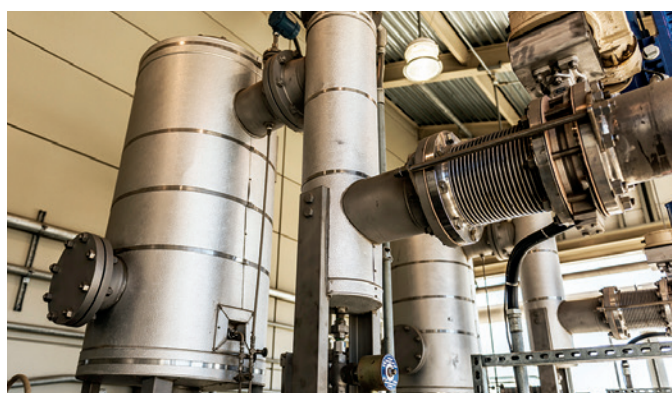
F.E. Weymouth Water Treatment Plant Ozone destruct unit
