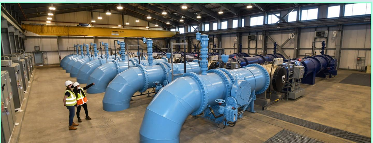
LADWP engineers inspect some of the 15 UV reactors at the LARUVDP designed to provide high-quality drinking water.
