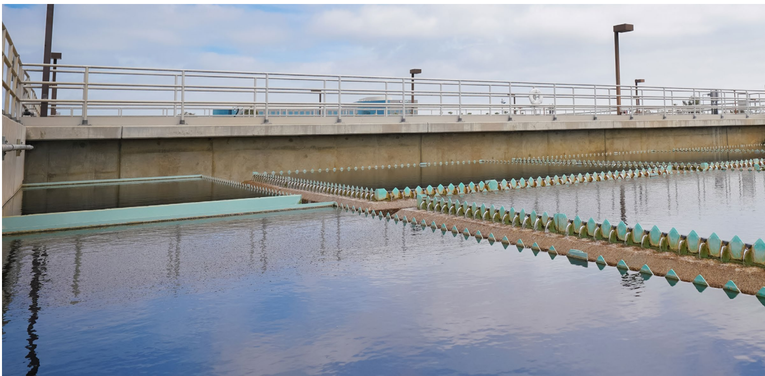
Pictured: Drinking water pools at the Groundwater Treatment Plant going through the sedimentation basins before entering the filtration process
