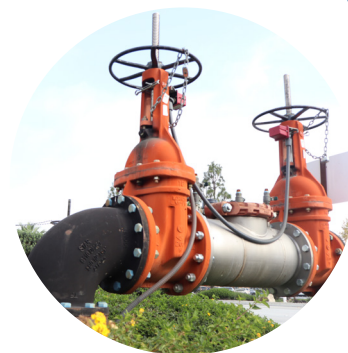
Double Check Backflow Prevention Assembly
