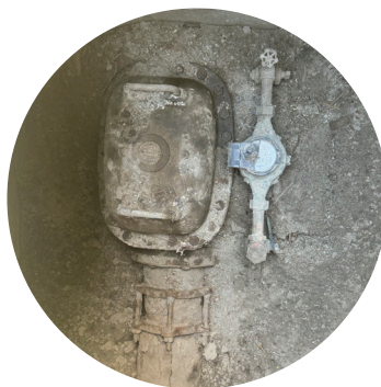
Single Check Backflow Prevention Assembly
