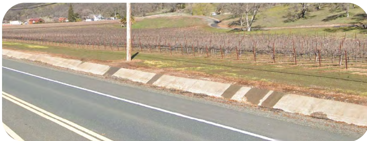
Figure 5.2.2 Concrete Drainage Channel in Clearlake Oaks (along north side of Hwy 20)
