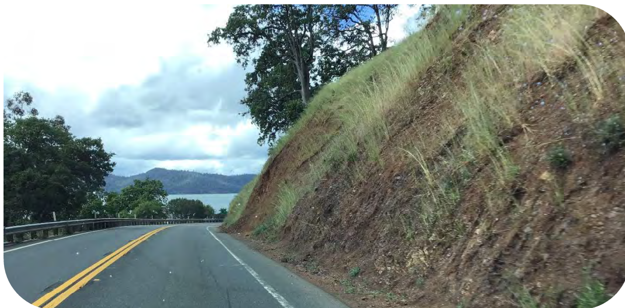
Figure 3.5.2A- Typical Erosion at the Cut of a Slope along Highway 20
