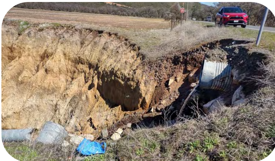
Figure 3.5.2B- Example of Severe Erosion on Nearby Highway 29 South Of Clear Lake
