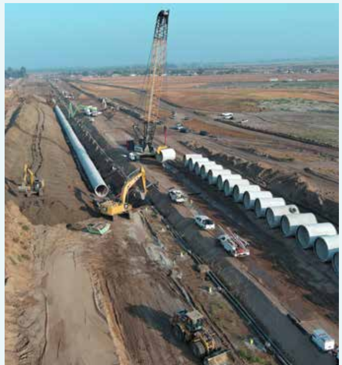
Contra Costa Water District recently replaced the beginning section of the Contra Costa Canal with a 10-foot diameter pipeline. This project improves public safety, water supply resiliency, and water quality.
