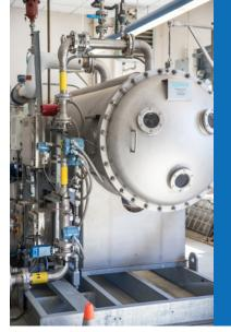
The use of ozone disinfection results in drinking water that is very safe, with little taste and odor. Ozone effectively destroys potentially harmful microorganisms and, by breaking up the organic material often found in water, vastly improves the taste and odor of drinking water. In addition, ozone disinfection reduces the formation of many disinfection byproducts, such as trihalomethanes, a class of suspected cancer-causing compounds associated with chlorine disinfection.
