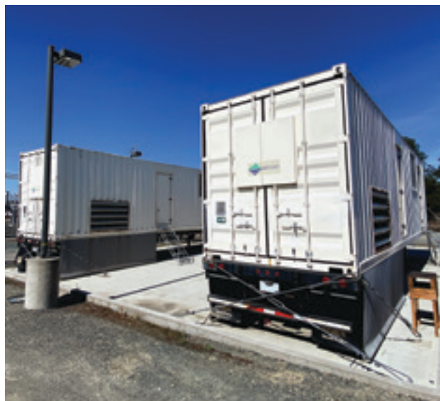
Backup generators would keep our water treatment plants running during an emergency.
