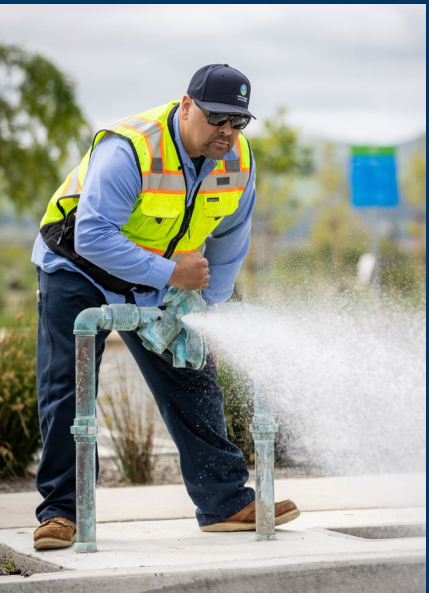
A DSRSD employee opens a test cock on a backflow prevention device to verify that it is receiving water flow.
