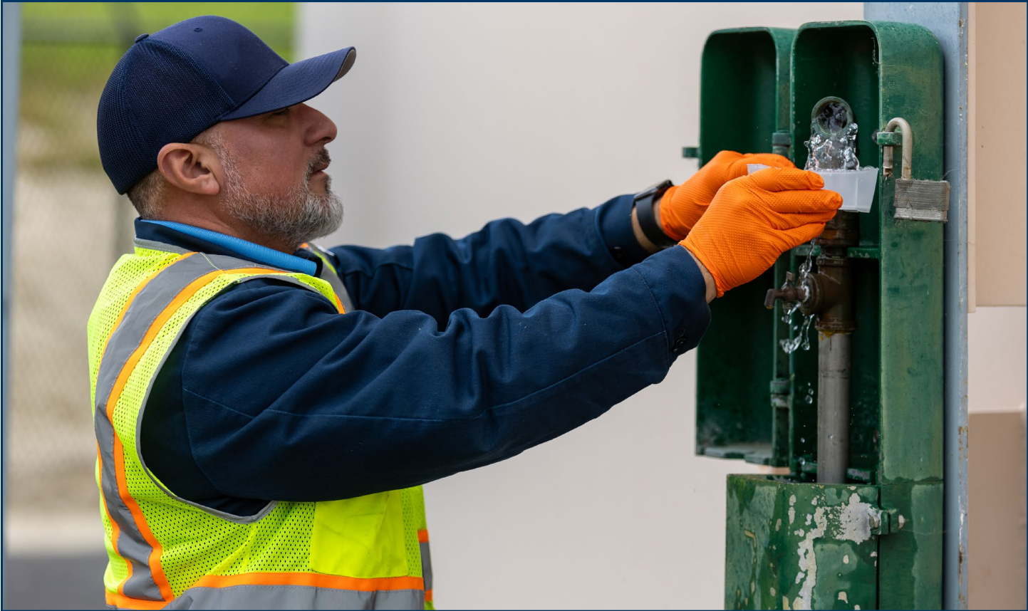
A DSRSD employee takes a water sample from a reservoir. All drinking water reservoirs are sampled once a week to ensure water quality throughout the system.
