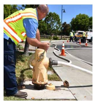
Water Systems Lead Operator Danny Leonardo opens a hydrant used to flush a drinking water main at the end of Trescott Court in Dublin. Flushing water lines is one of the best ways to improve water quality.
