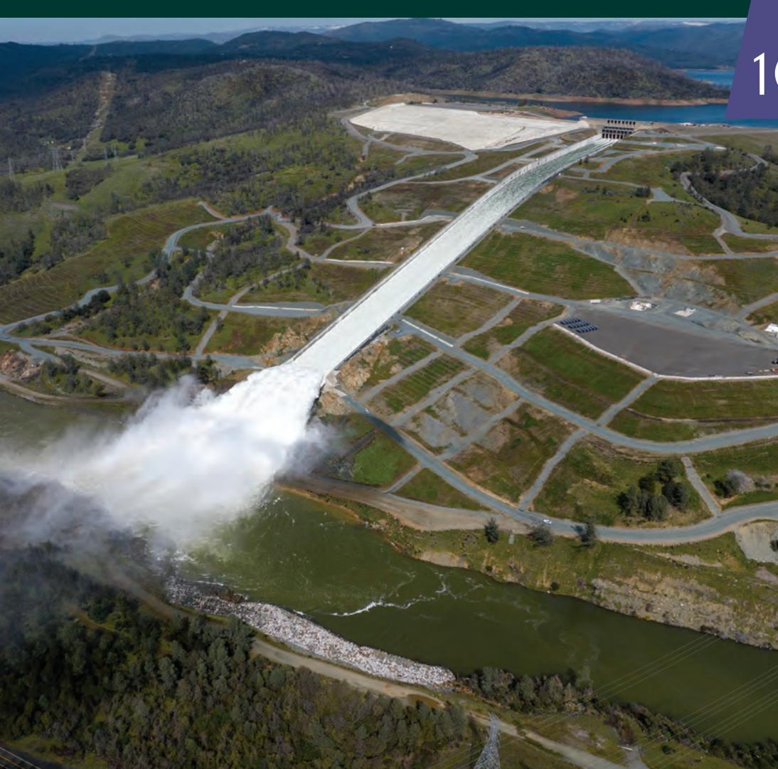
*A drone aerial view of a cloud mist formed as water flows over the four energy dissipator blocks at the end of the Lake Oroville Main Spillway. Photo taken March 17, 2023.*
